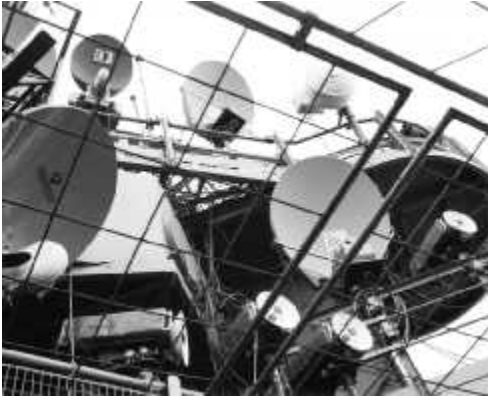
Microwave antennae on the top of the Eiffel Tower in Paris. (E.H.)
